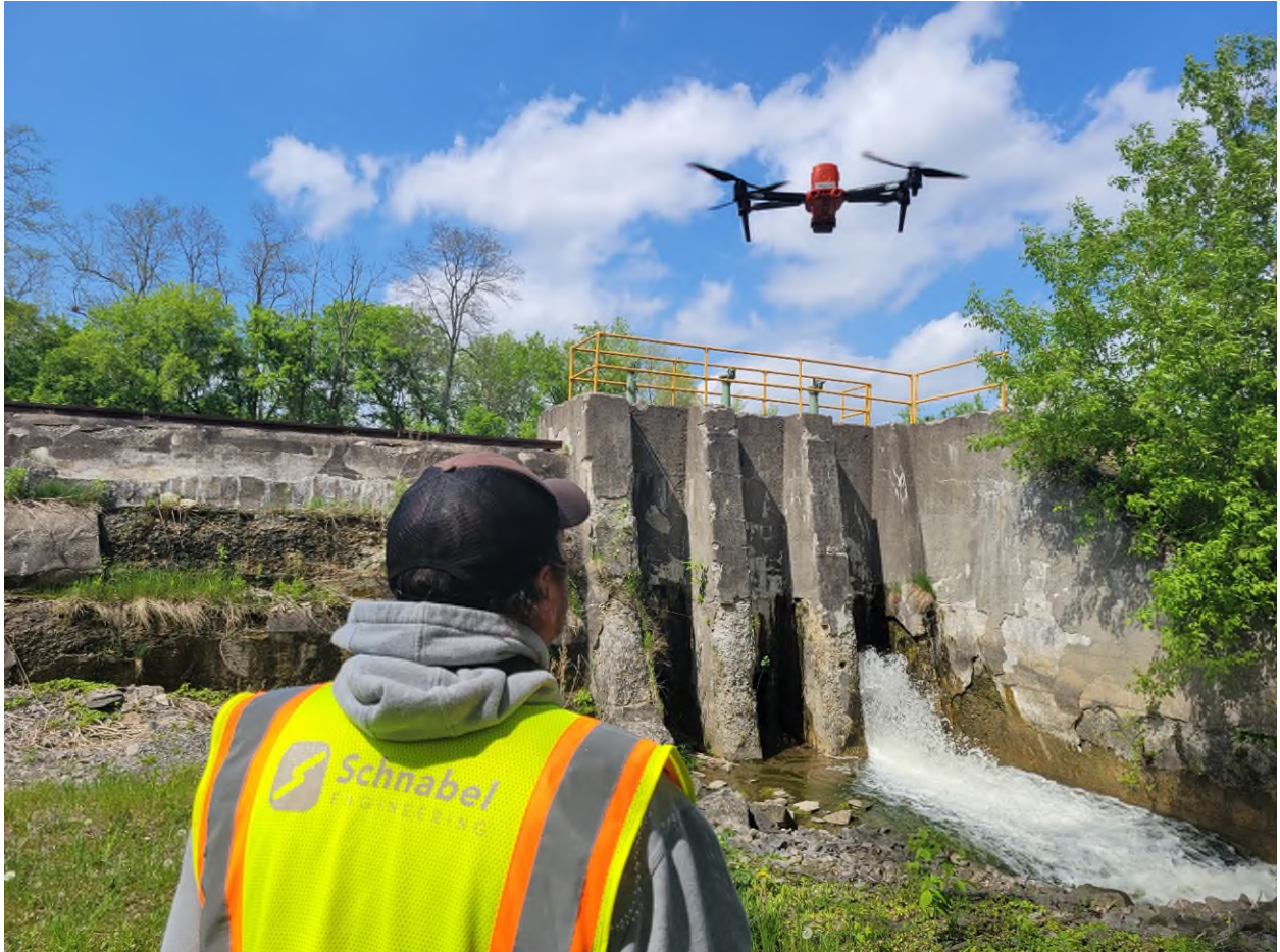
Example photo of drone inspection
